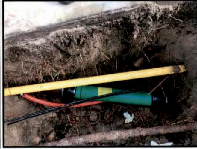
(FIOS) Lateral Repair 418 Locklie Street
