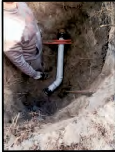
(FIOS) Main Line Repair 509 Wilkie Street
