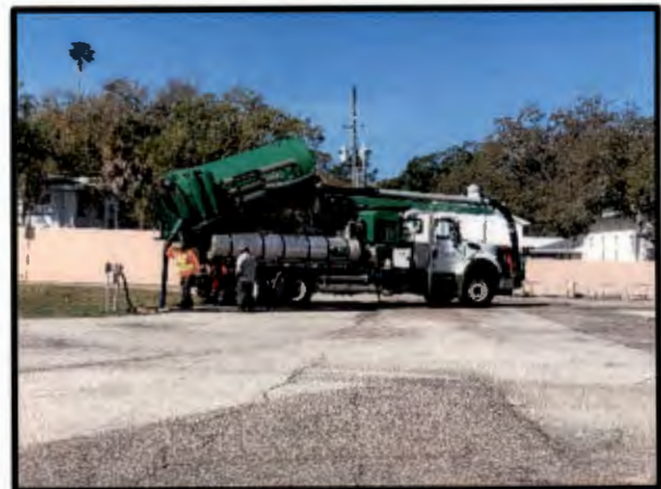
Decanting at the Wastewater Treatment Plant
