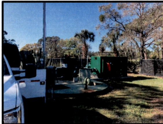
Maintenance on Lift Station #8
