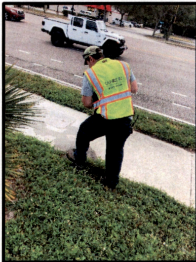
Water Service Repair 1804 Main Street
