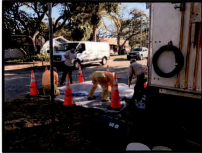
R/E Liner Install Broadway
