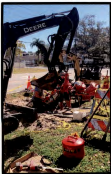
Fire Line Repair 880 Patricia Avenue
