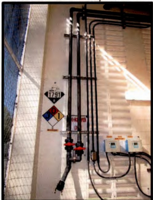
Replaced both 2" Bleach Tank Fill Lines
