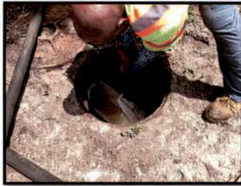
Finish cutting of new liner
