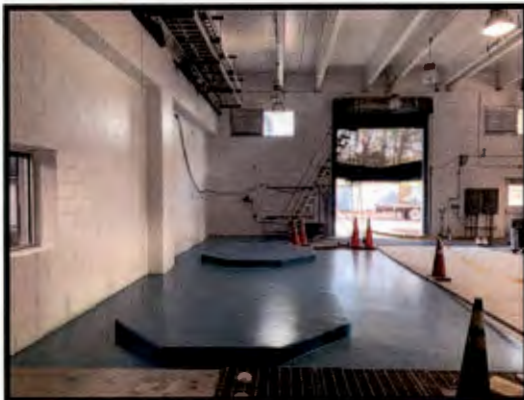
CIP Pads and Floor Coating
