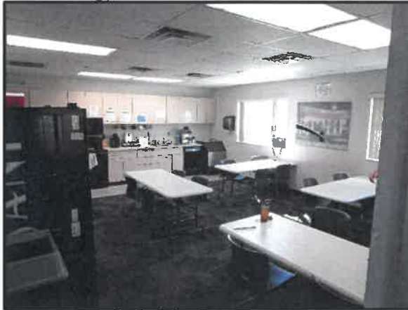
New Floor Tile/Carpet and Walls Painted In the Breakroom
