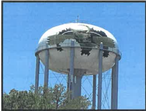
Artwork on the east facing tank side
