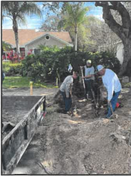
Potable Water Meter Relocation 1061 Weathersfield Drive
