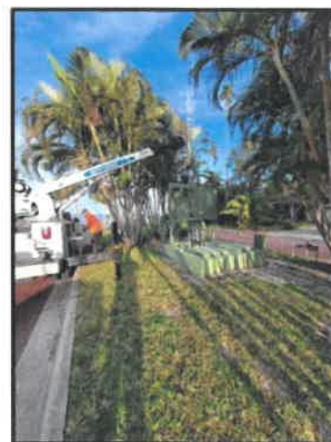
LS #4 Pump Replacement
