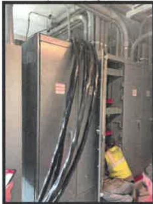
Large Gage Wire Installation
