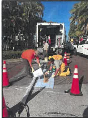
Liner Install LS #4
