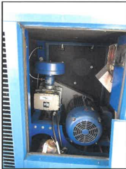
FET Blower #2 Installed New Blower
