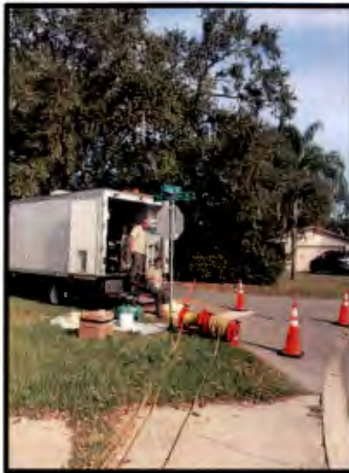
San Christopher Drive and Keene Road Main Line Liner Installed
