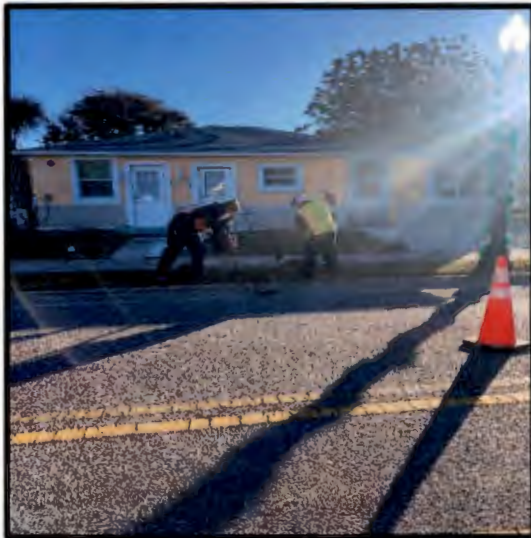
Waterline Repair 437 Douglas Avenue
