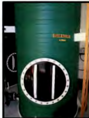
New Access Hatches on Sodium Bisulfite Tanks Fac #14B
