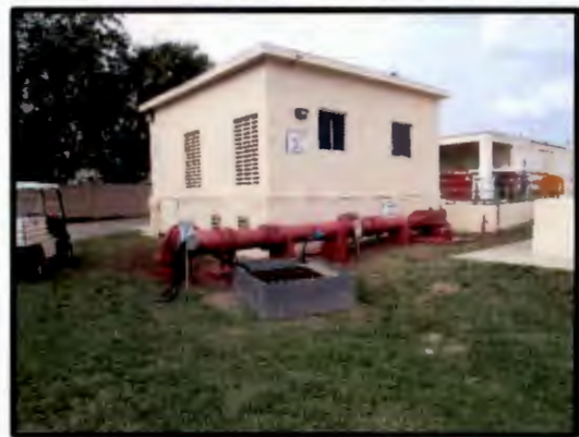
Staff painted external Master Reuse Piping at Fac #16
