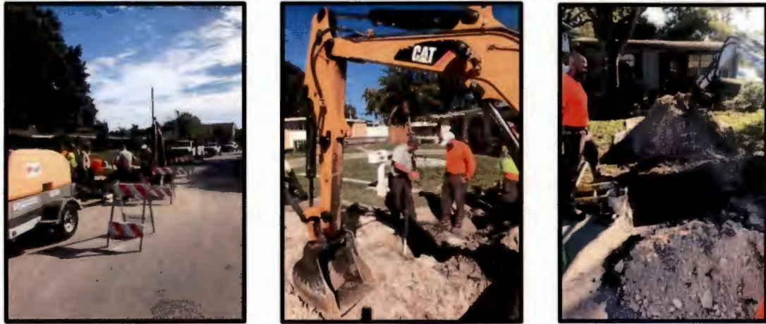
566 Baywood Drive South Lateral Liner Installed
