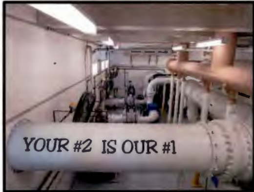
Fac #8 Filter Building Fans x3 Installed for Circulation
