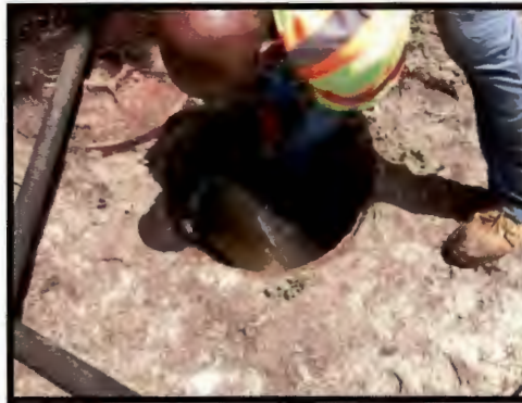
Finish cutting of new liner
