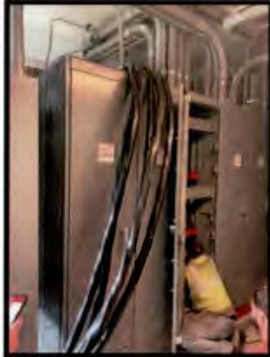
Large Gage Wire Installation
