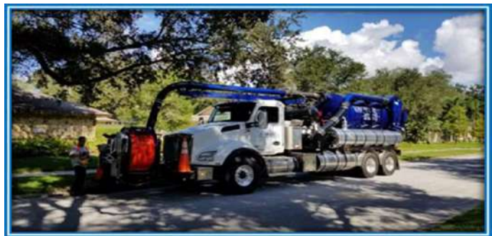
Stormwater Outfall Construction
