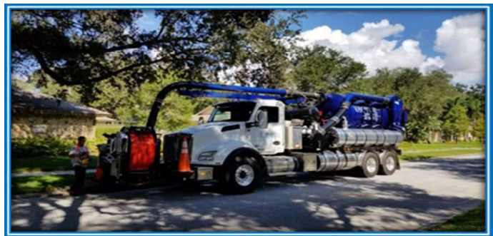
Stormwater Outfall Construction
