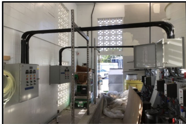
Reverse Osmosis Water Treatment Plant - Reconstruction / Restoration Project
