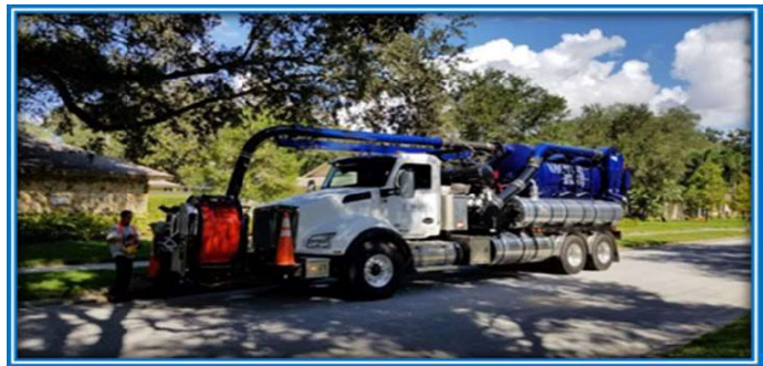
Stormwater Outfall Construction
