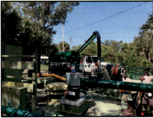
Lift Station #8 Cleaning
