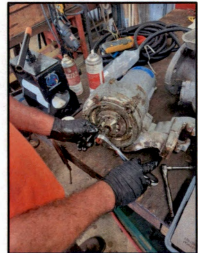
Pump Repair Lift Station #40
