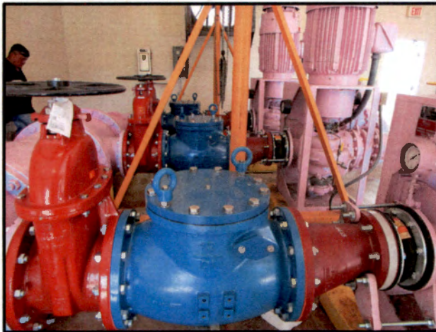
Belcher Road Valves and Check Valves Replaced Administration Building
