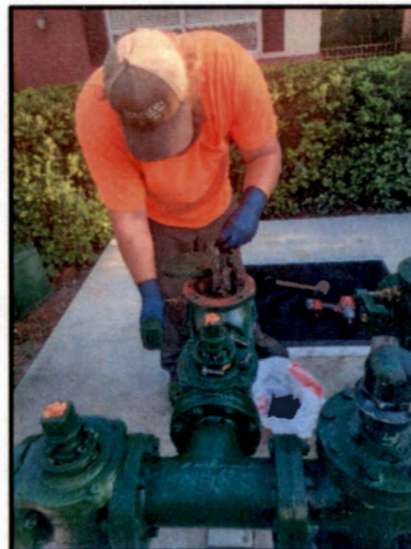
Cleaning Check Valve Lift Station #12A
