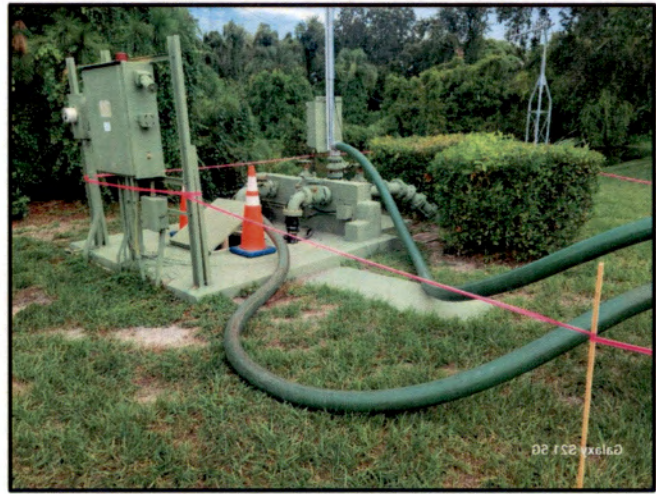
By-pass Set-up at Lift Station #32
