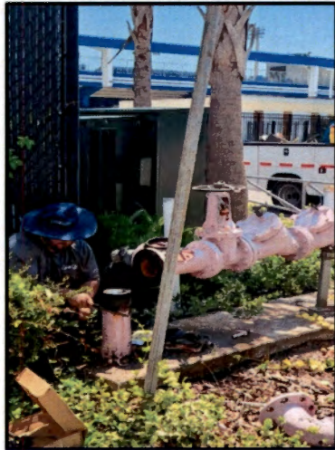
373 Douglas Avenue Large Reclaimed Meter Repair
