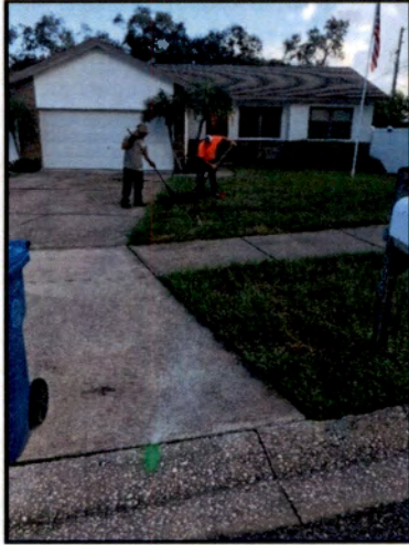
Clean Out Install 1608 Coastal Place
