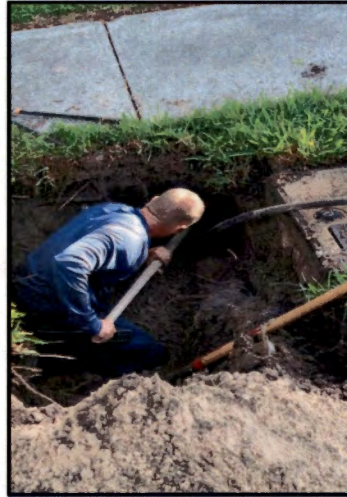
2254 Harbor View Drive South Potable Service Line Repair
