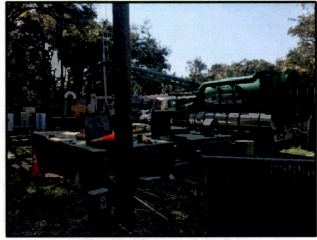
Lift Station #10 Cleaning
