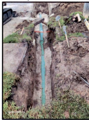
Main Line Repair 1181 Dinnerbell Lane East/South
