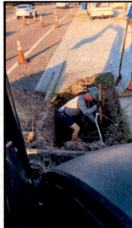
Water Line Service Repair 632 Main Street
