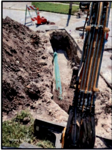
Main Line Repair 1181 Dinnerbell Lane East/South
