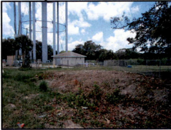
New Fencing and Swing Gates Installed Curlew Reclaim Tank
