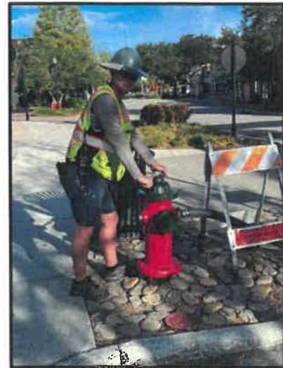
Install Hydrant Meter Main Street / Pinellas Trail
