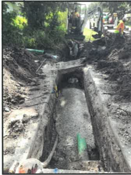
Main Repair James & Vine
