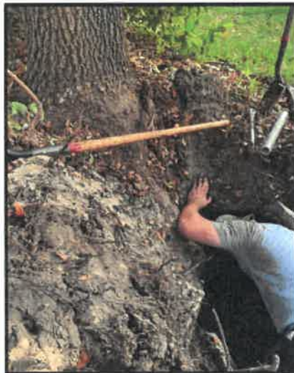
Potable Water Service Line Repair 269 Ashley Court
