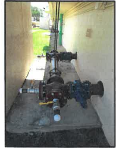
New Isolation Valves Installed Between Digester #3 & #4 Fac
