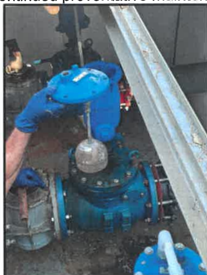
ARV Repair Lift Station #15
