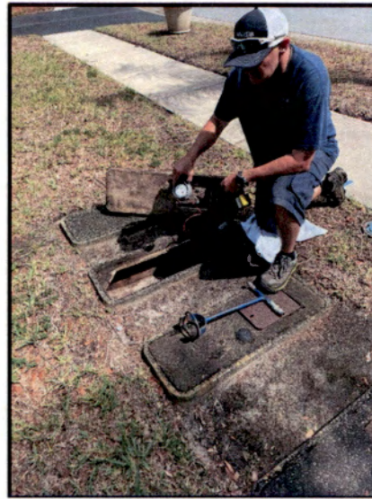
Water Service Line Repair 1800 Main Street
