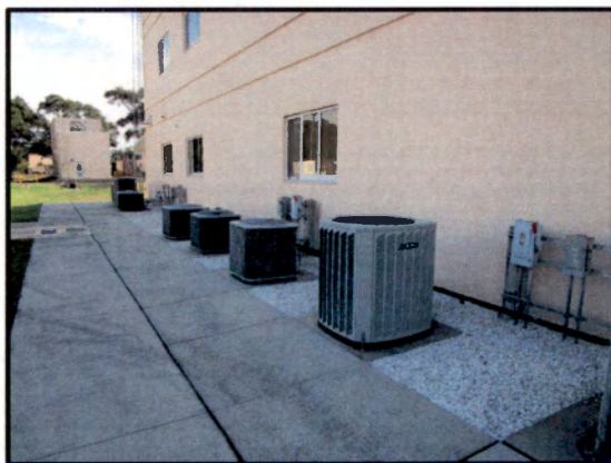
New Shell Around Facility #2 Admin Building
