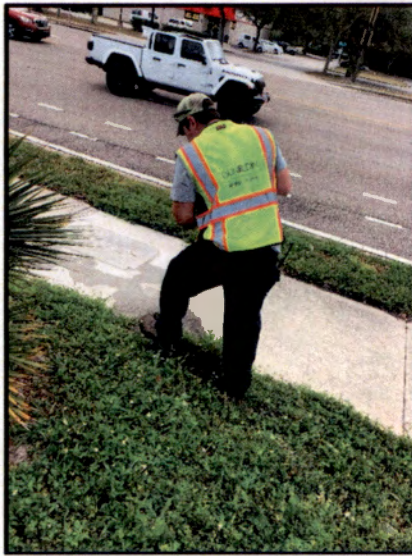
Water Meter Register Changeout 1585 Amberlea Drive South
