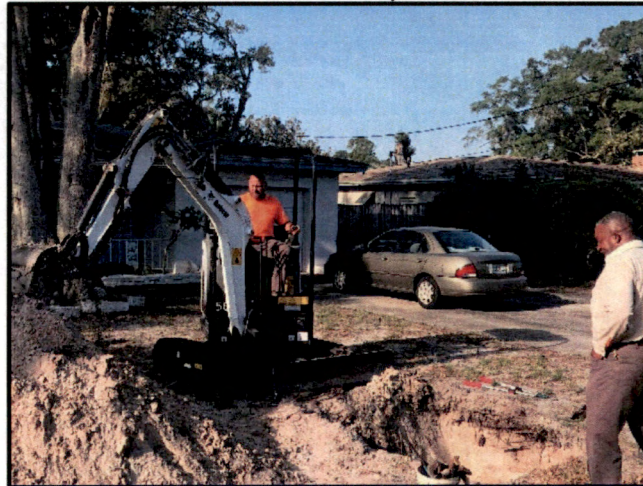
Lateral Repair 947 Virginia Street
