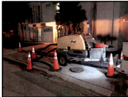
By-pass for Main Street Lining on Milwaukee Avenue
