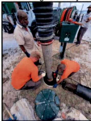
Cleaned Wet Well & Installed New Floats LS #44
