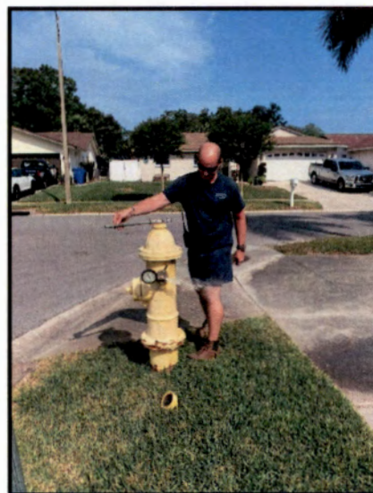
Fire Hydrant Maintenance 1605 Amberlea Drive South
