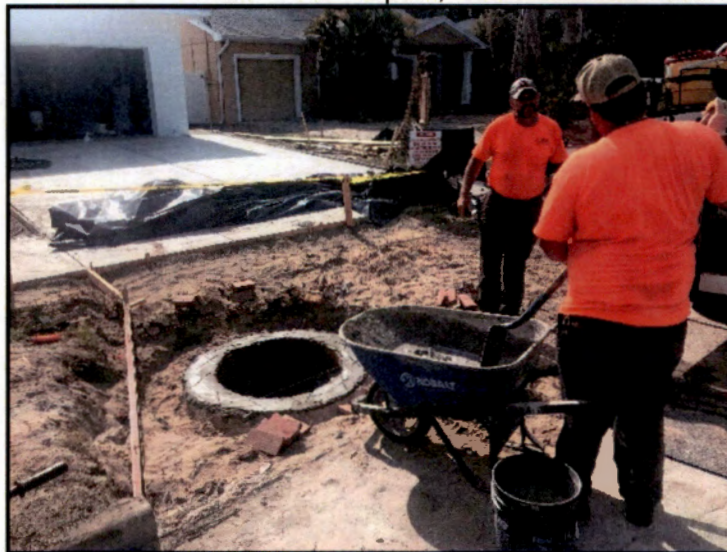
Manhole Repair, 39 Broadway
