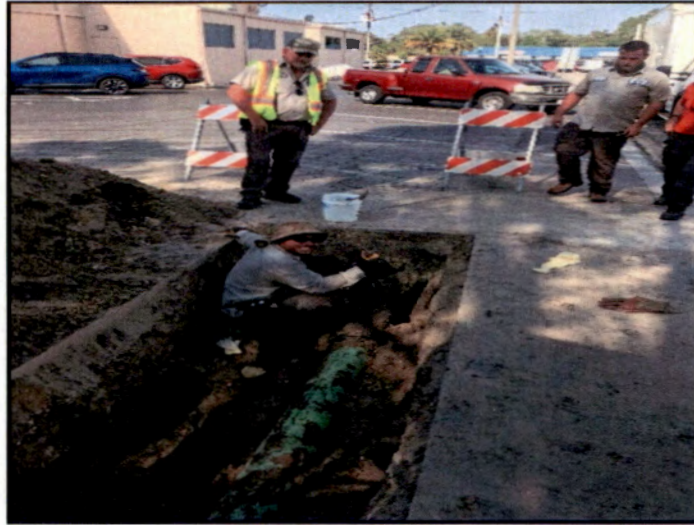
Main Line Repair, 405 Patricia Avenue
