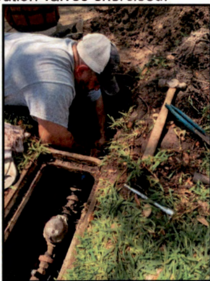
Potable Water Service Repair 750 Kirkland Circle
