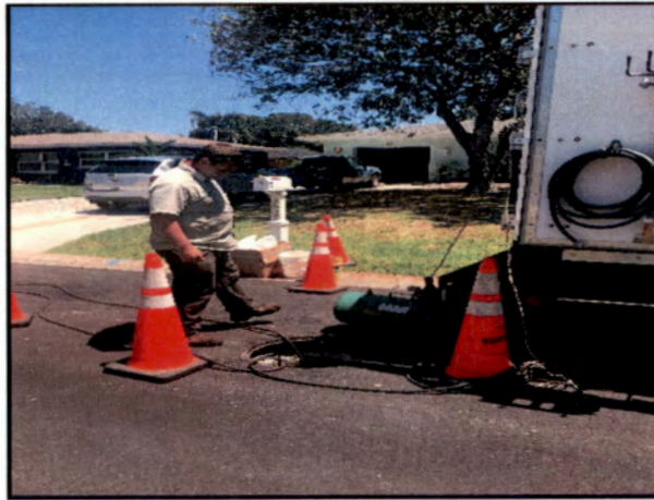
Installed Sectional Liner 83 Oakwood Drive
